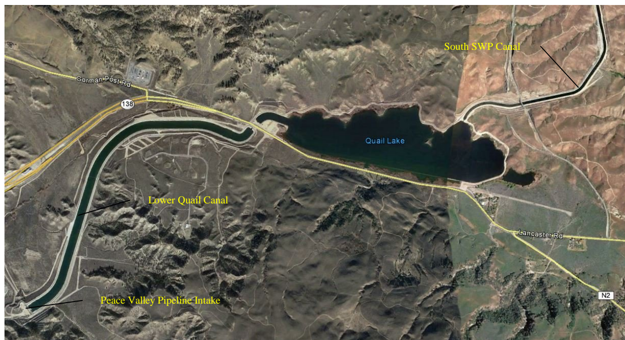
Figure 2. Aerial view of Quail Lake (Source: staff).
