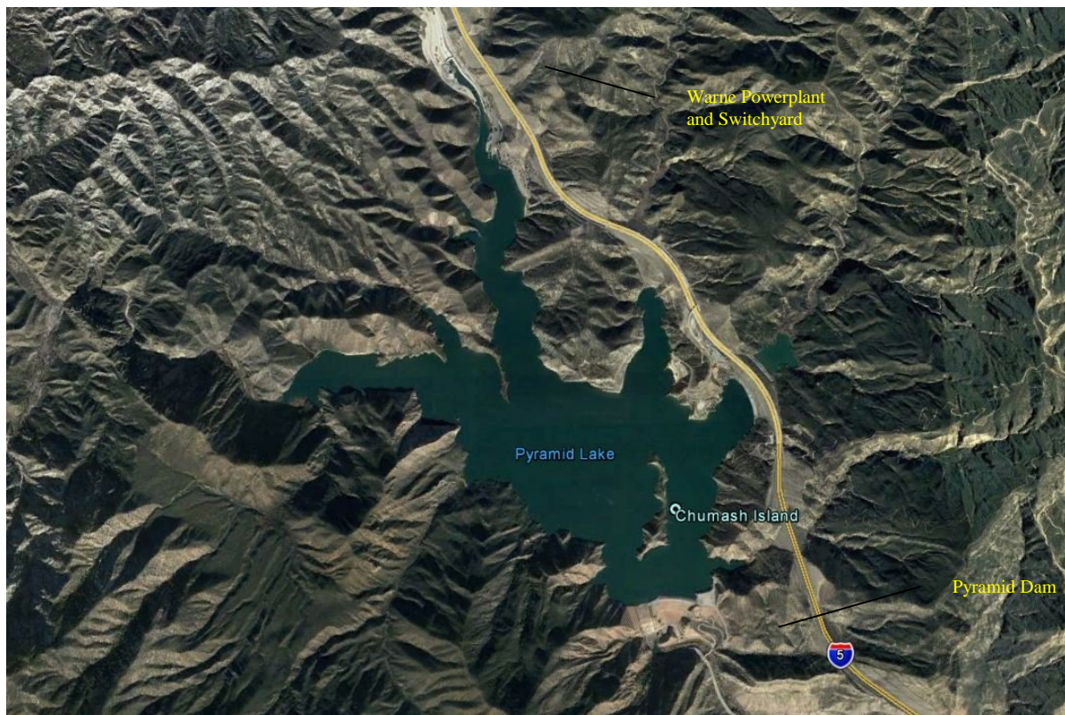
Figure 3. Aerial view of Pyramid Lake, Warne powerplant, and switchyard (Source: staff).
