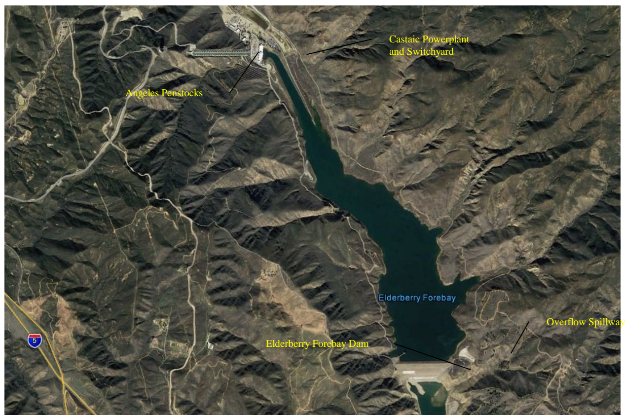
Figure 4. Aerial view of Elderberry forebay, Angeles penstock, and Castaic powerplant (Source: staff).
